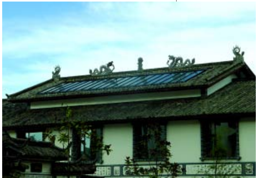
Rooftop solar hot water systems on a restaurant in Lijiang. © Photo courtesy of Li Junfeng.
