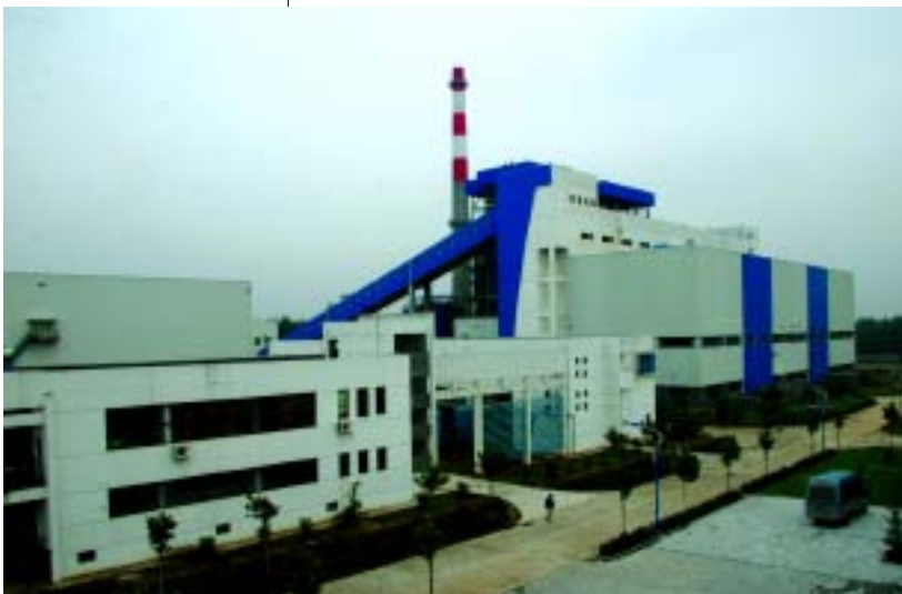
Biomass power plant in Jinzhou, Hebei province. The plant's primary feedstocks are corn and wheat stalks and tree branches.
